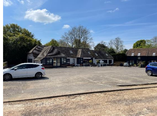
Figure 7 - Alfold Business Centre to southwest of site
