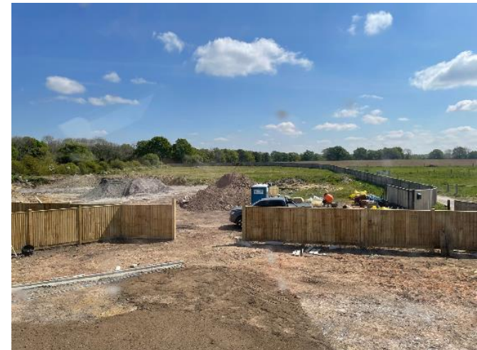
Figure 4 - View of site from neighbouring site to west
