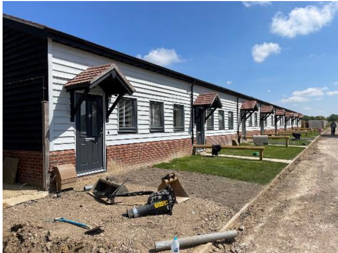
Figure 6 - New dwellings to west of site
