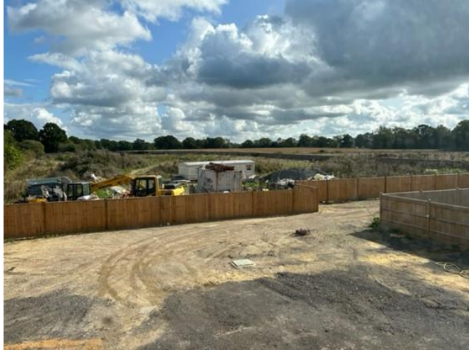
Figure 5 - View of site from west(site beyond far fence)
