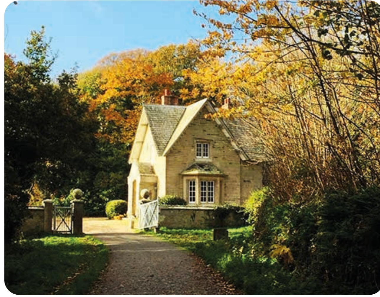
Example of a village gatehouse nestled in woodlands
